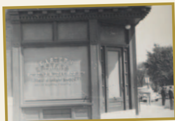
Eastern Building and Loan Society at 701 N. Milton Avenue
